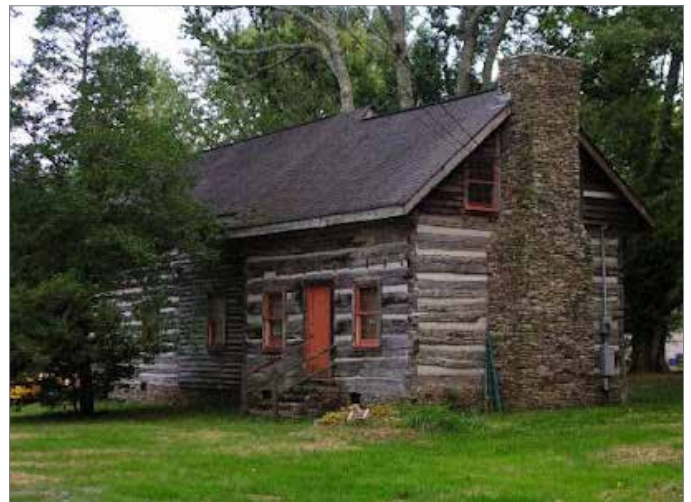
The Toll House Source: Waymark
