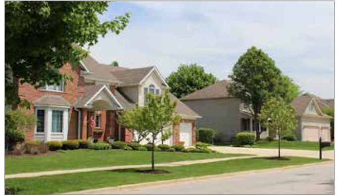
Residential Example Source: Marco Homes
