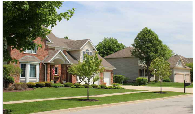
Residential Example Source: Marco Homes
