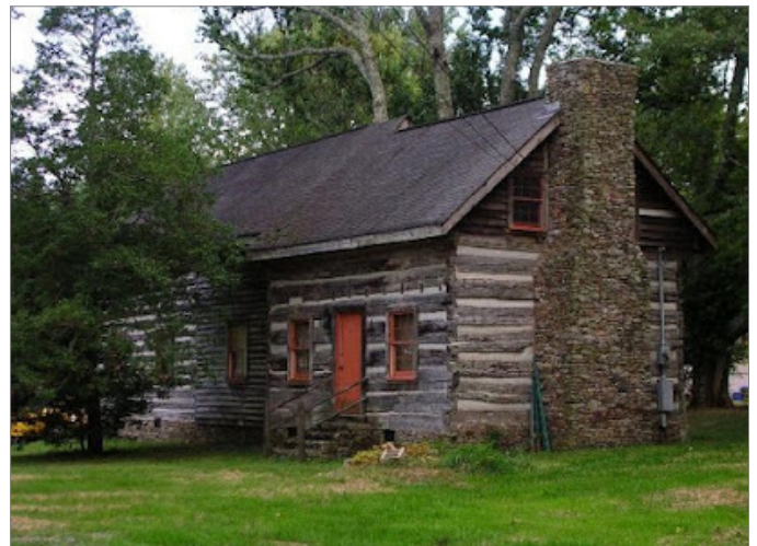
The Toll House Source: Waymark
