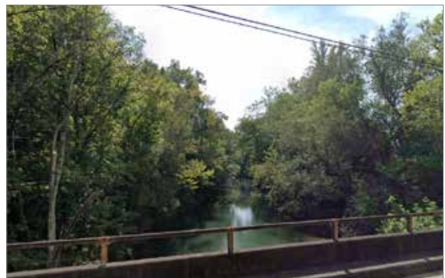
North Chickamauga Creek & Boy Scout Road (Floodway Zone) Source: Google Earth
