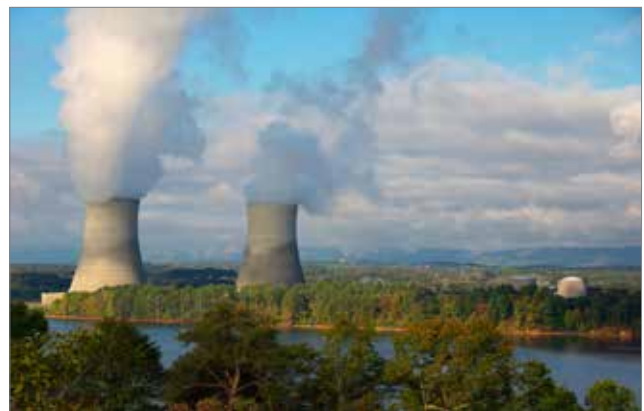
Sequoyah Nuclear Plant Source: After Action Report, FEMA
